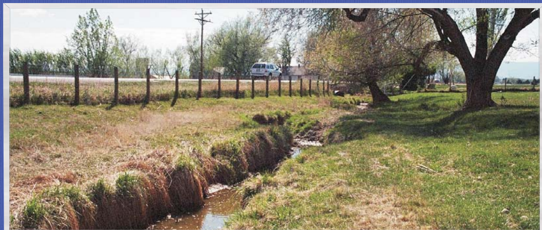
Irrigation ditch A, north of SH 402
