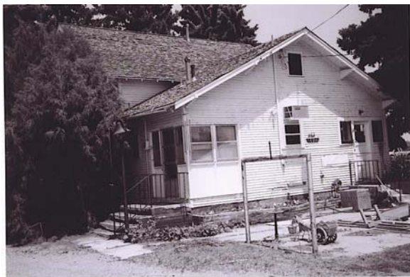
Main House: rear elevation, view to northeast
